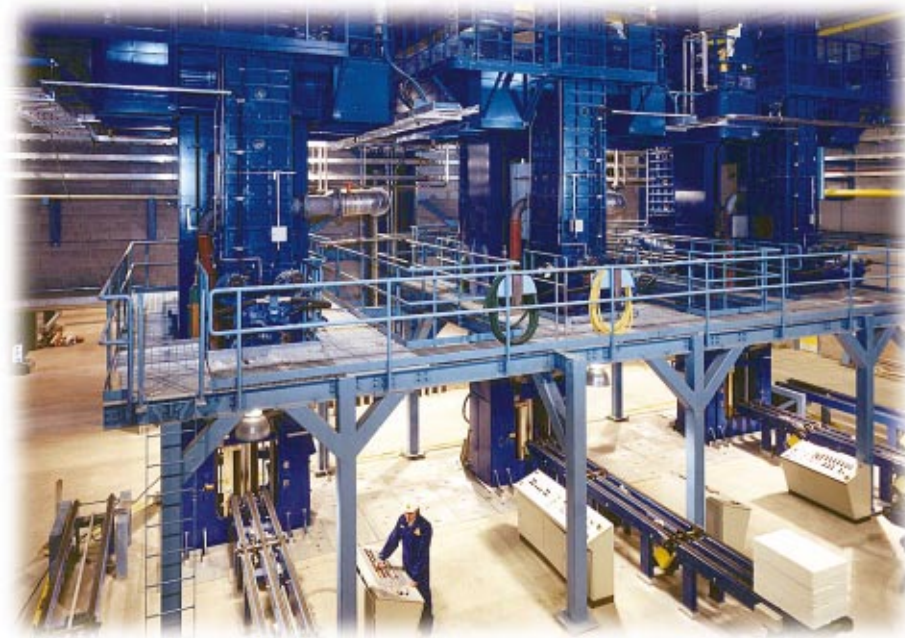
Millar Western's slab presses are high-production machines that apply 400 metric tons of force with a large vertical stamp, three or four times through each cycle.
